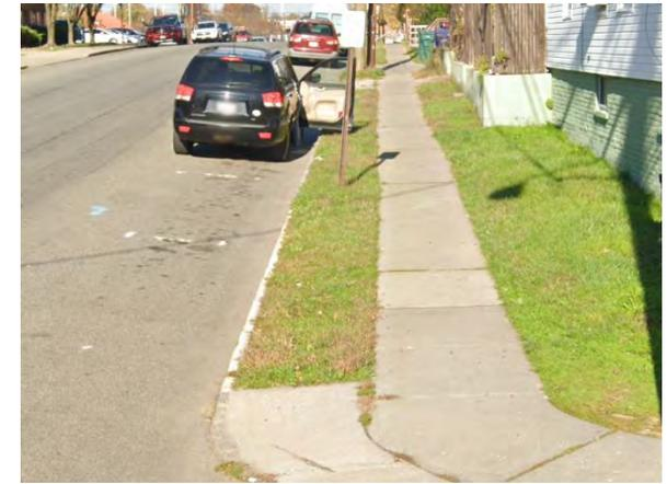
The grass strip on the east side of 2nd street, north of Gordon Street, can be converted to a stormwater planter to capture, treat, and infiltrate the stormwater runoff from the roadway. A preliminary soil assessment suggests that more soil testing would be required before determining the soil's suitability for green infrastructure.
