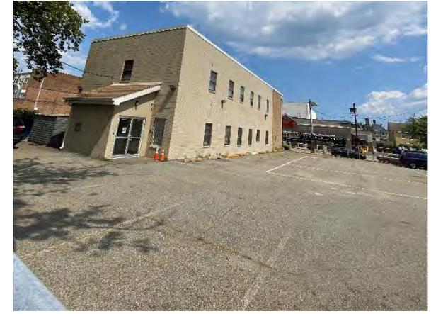
The existing planter bed can be converted to a rain garden to capture, treat, and infiltrate the stormwater from the existing downspout. A section of the parking lot spaces in the southeastern corner can be converted to pervious pavement to capture and infiltrate the stormwater runoff from the parking lot. A preliminary soil assessment suggests that more soil testing would be required before determining the soil's suitability for green infrastructure.
